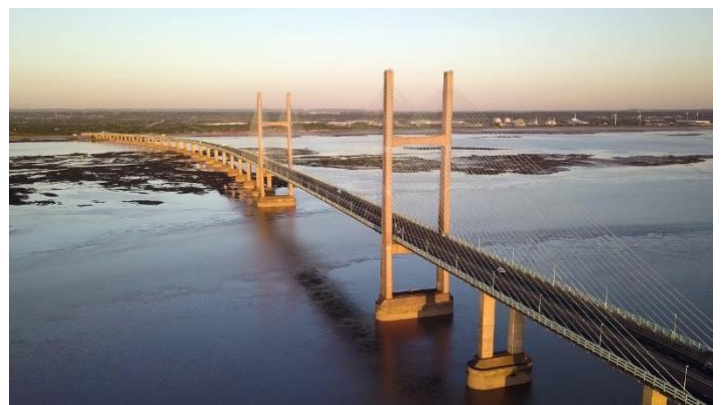
Prince of Wales Bridge
